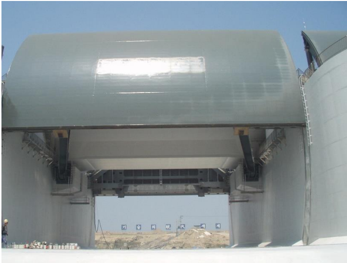
Figure 7.4. Garyeok Sluice gate constructed on island, 50x30m
